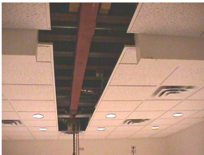
Figure 9.2 Properly installed false ceiling with I-section girder
